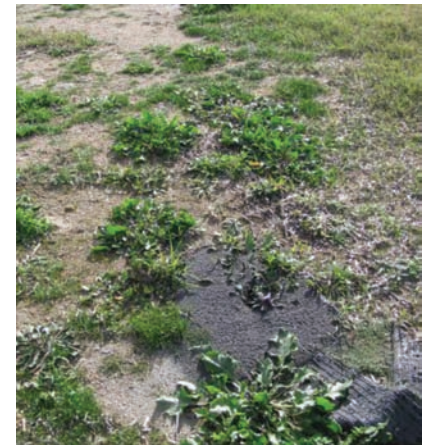
Figure 16. Spots of sea sand that was ejected during soil liquefaction caused along a ground crack opened to the south of Lixouri port with the first strong earthquake.
