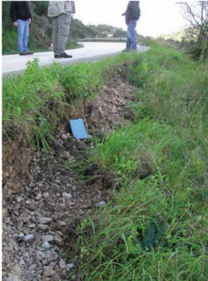
Figure 13. Landslide caused downslope in the road at the foothills of Mt Vlikatari to the SW of Myrtos, NW Cephalonia, with the first strong earthquake of 26.1.2014.
