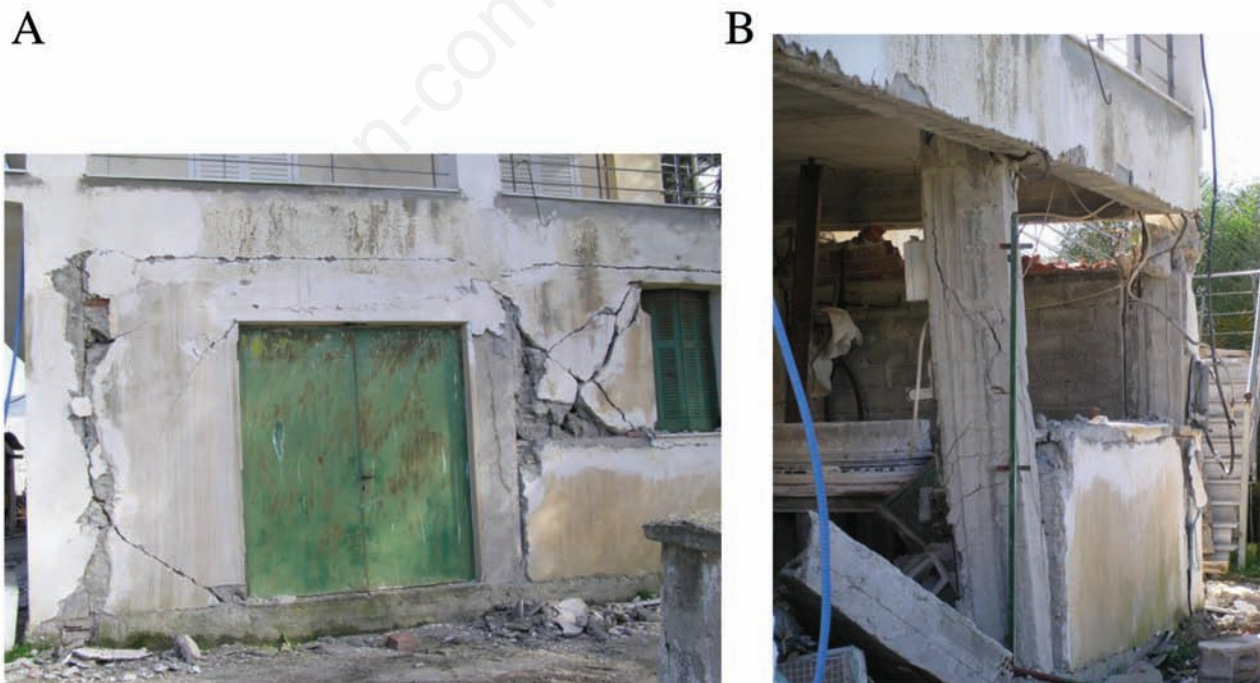
Figure 10. Example of two-storey building in Ayios Dimitrios village (see location in Figure 9) damaged by the first (A) and the third (B) Cephalonia strong earthquakes.
