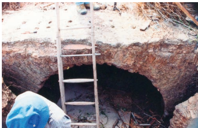
Figure 1. Kiln CD near the town of Castelo de Vide. The perforated floor of the firing chamber, and the underlying combustion chamber, are clearly visible. The basal part of the next arch supporting the (now removed) continuation of the firing chamber floor is visible in the lower right.
